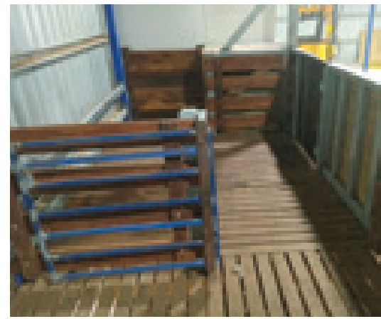
The catching pen, with slats running to the board. The boards run across the flow of sheep in both the catching pen and the fill pen reducing the light visible below the shed as sheep move through.
